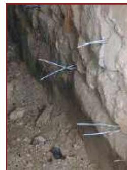
10. Follow same procedure for all cross-links in walls
