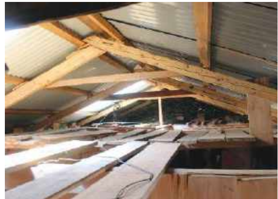
R.3.2 Connection of wooden truss
