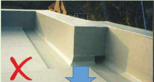
URM masonry parapet wall
