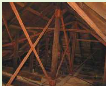
Steel bracing to roof
