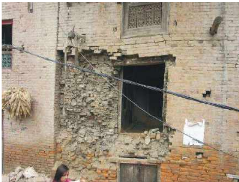
C.4.2 Low strength masonry : BMM
