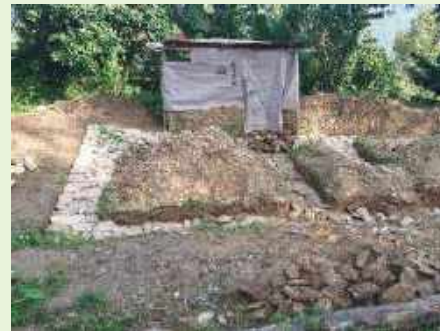
Insufficient foundation
