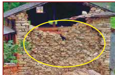
Delaminated wall
