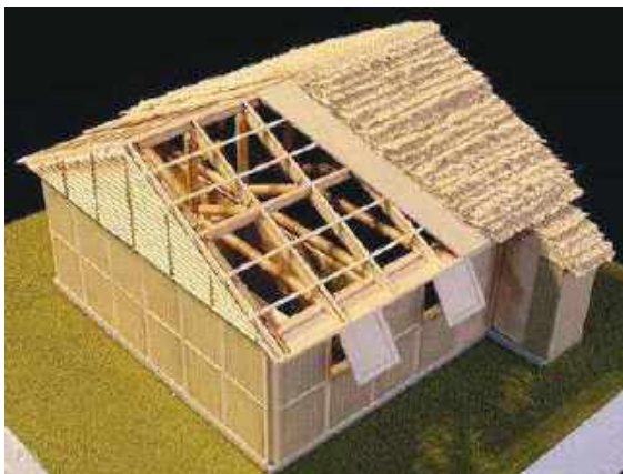
R.3.3 Bracing missing in inclined roof
