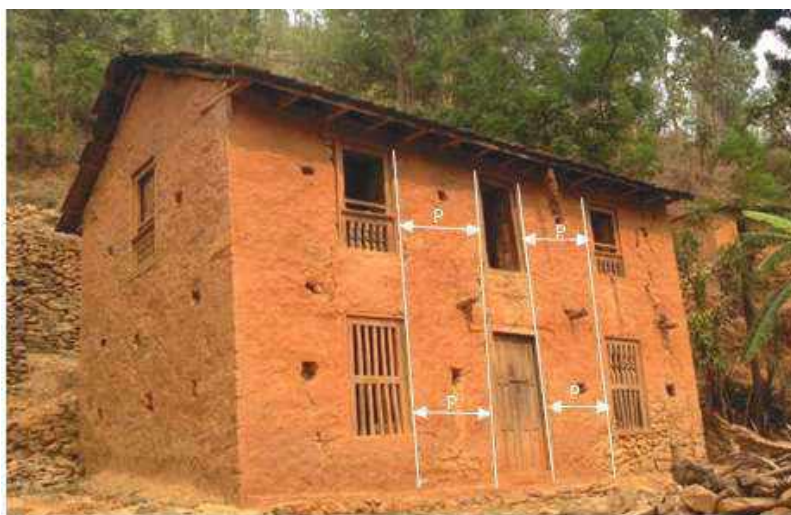
Figure 1-5 Photo depicting pier lengths
