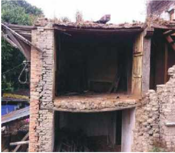
R.6.1 Damaged buildings showing wall-to-floor(joist) connection in Bungamati
