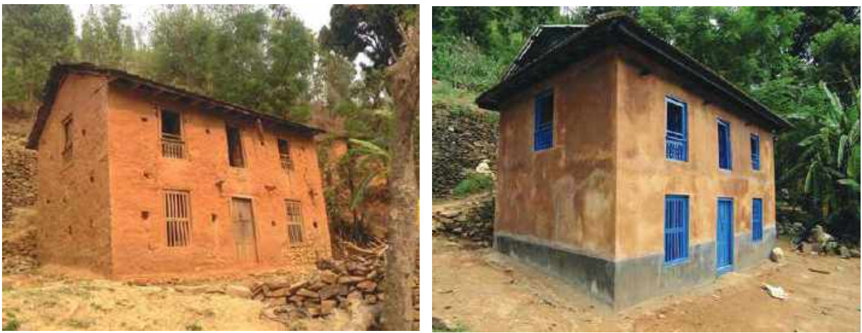
Figure 1 SMM house before and after implementation of Standard Type Retrofit
