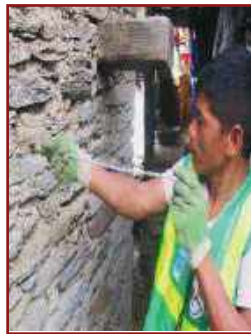
5. Insert cross-links in the holes at pre-determined location on walls.
