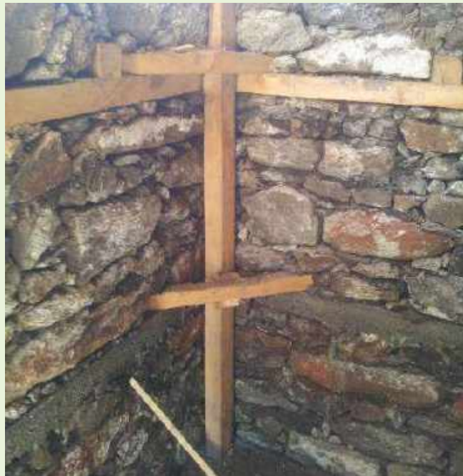
Installation of wooden vertical member from inside of the wall
