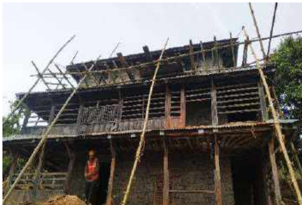
Figures 18 & 19: Splint & bandage approach retrofitted houses Left: ongoing retrofitting; Right: after retrofit
