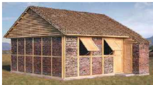
Use of timber planks at Gable part
