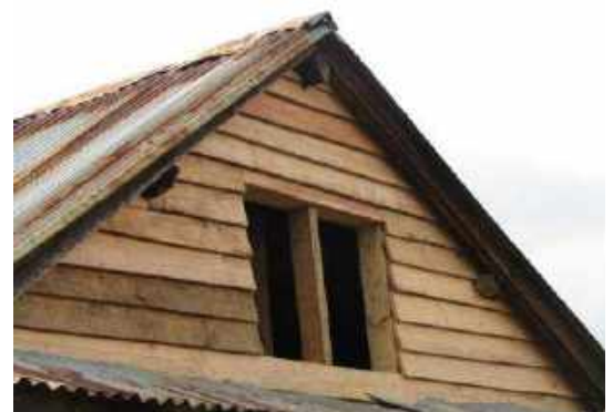
Figure 12: Light gable (Photo credit: Build Change)
