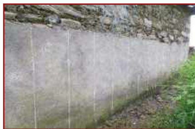
Marking of vertical CR wires on walls
