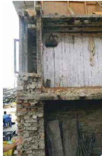
R.6.1 Damaged buildings showing wall-to-floor(joist) connection in Bungamati
