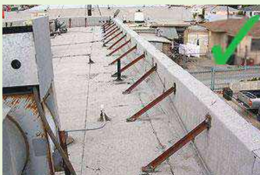
Masonry parapet braced with steel section with proper connection with slab or beam
