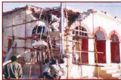
Cracked arcade being restored stone by stone.
