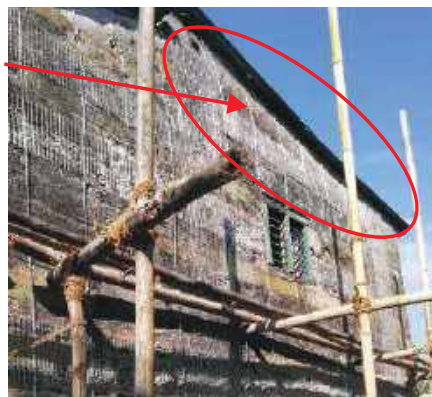
CR vertical wires going over gable
