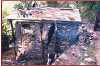
Undamaged RC slab on severely damaged wall
