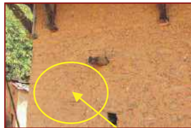
Wall having Grade 1 cracks
