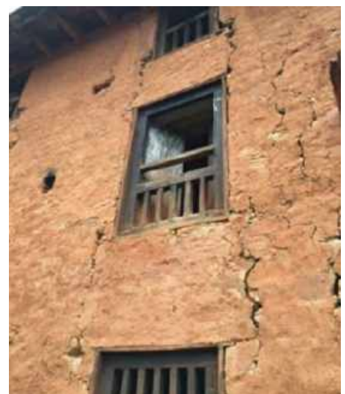
Figure 6: Diaphragm deficiency
