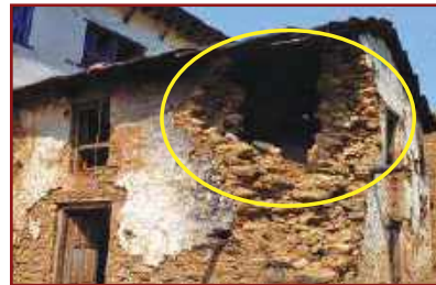
Collapsed corner
