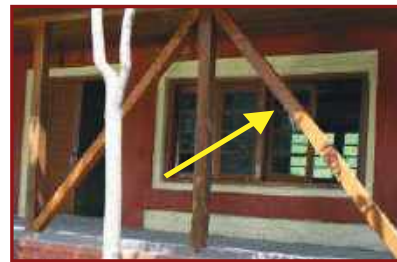
Alternatively, diagonal wooden bracings between column can be installed if space permits.
