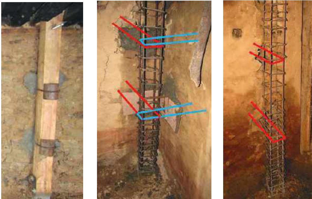
Figure 4-5 From left: timber strongback (typical at midspan of transverse walls); reinforced concrete corner strongbacks; reinforced concrete mid-wall strongbacks (typical along longitudinal walls)
