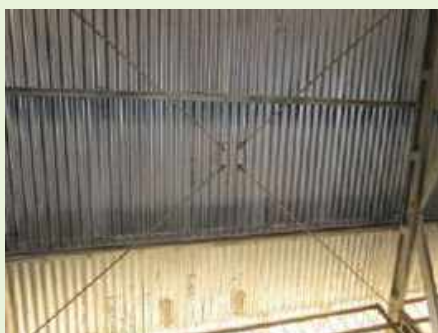
Diagonal Steel bracing to roof
