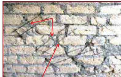
Install 8mm rebar with 100mm nails inserted with washer at staggered spacing no greater than 300mm.
