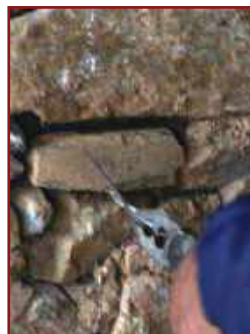
9. When pulled, cross-links should not come out without prying out the wedged chips.
