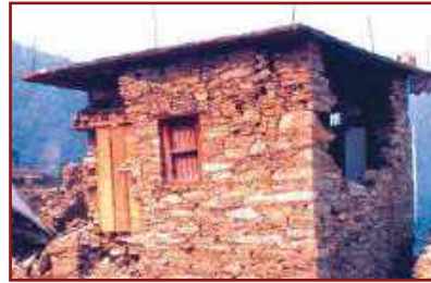
Undamaged RC slab on severely damaged wall
