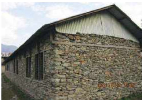
Use of C.G.I. sheet at Gable part
