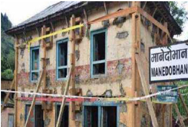
Figures 16 & 17: Strong back approach retrofitted houses Left: ongoing retrofitting; Right: after retrofit
