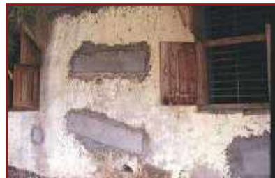
Plaster over the mesh with two 12mm coats of 1:3 cement mortar.
