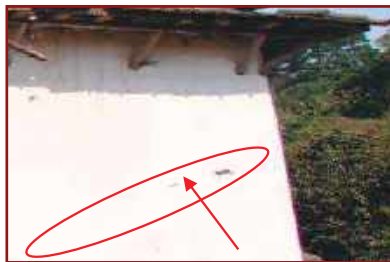
Wall having Grade 1 cracks
